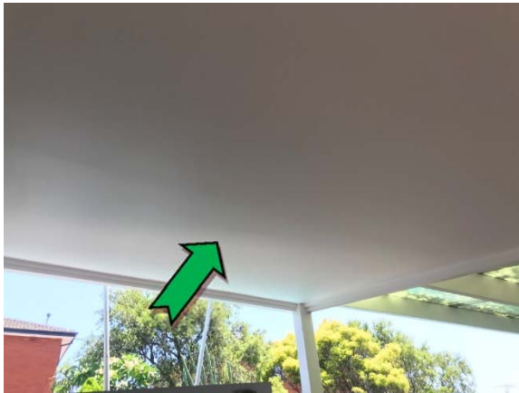
Photo 3. Exterior, shed, awning – non asbestos-containing fibre cement sheeting.
