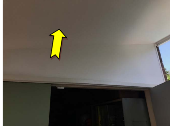
Photo 16. Exterior, awnings and high level infill panels – suspected lead-containing white upper paint systems.
