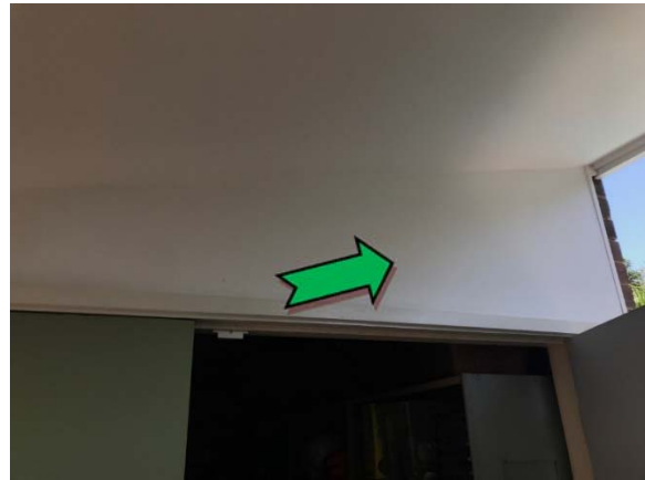
Photo 4. Exterior, shed, high level infill panel – non asbestos-containing fibre cement sheeting.
