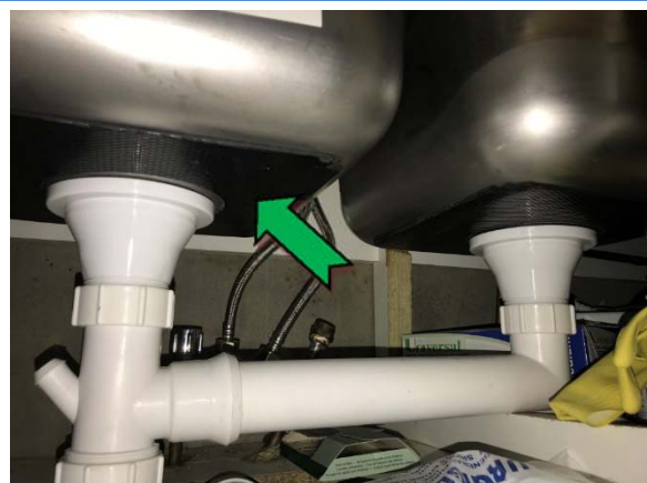
Photo 6. Interior, kitchen, under sink, sink pad – non asbestos-containing bituminous material.
