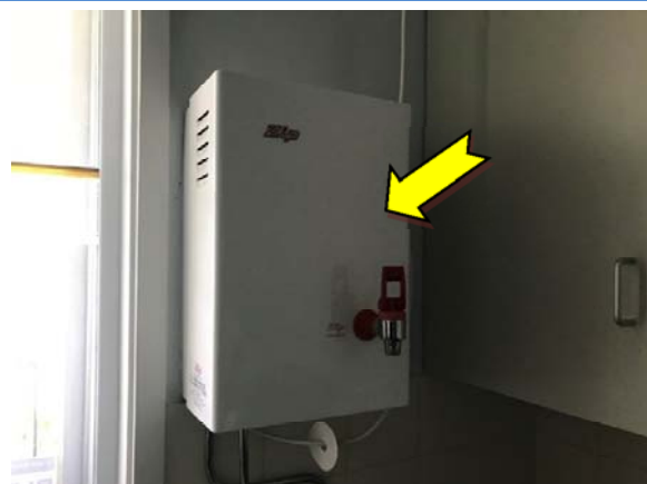
Photo 12. Interior, kitchen, hot water boiler – suspected SMF internal insulation material.
