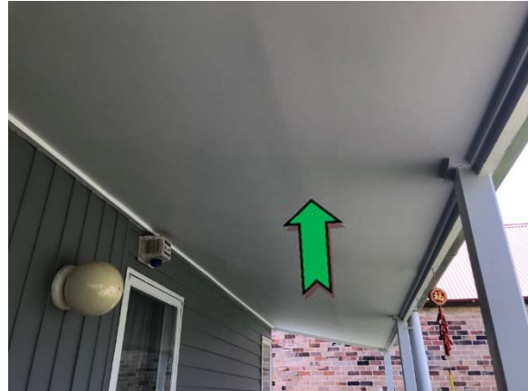
Photo 2. Exterior, east elevation, awning – non asbestos-containing fibre cement sheeting.
