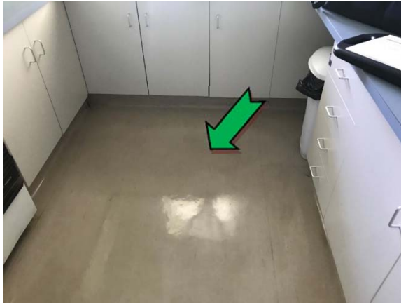
Photo 7. Interior, kitchen, floor coverings – non asbestos-containing sheet vinyl.
