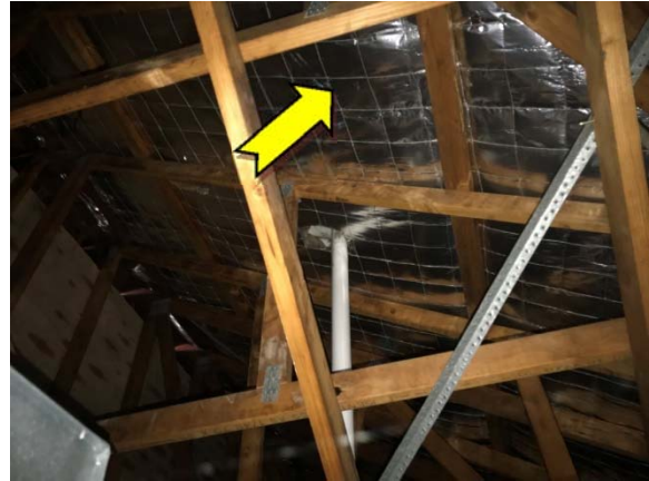
Photo 14. Interior, roof space, throughout – suspected SMF sarking insulation material.
